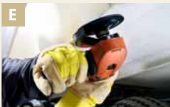
E Removing osmosis
