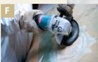
F Sanding out repairs
