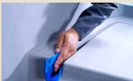
Preparation/repair of the negative mould
