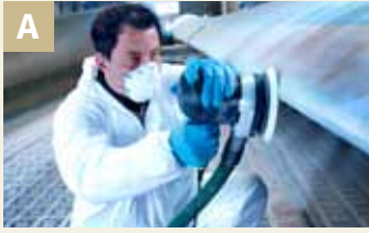
A Grinding edges after cutting
